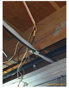
Electrical wiring was installed incorrectly. Non-metallic wiring should be installed in such a manner that it is not prone to damage. This is a safety hazard.
