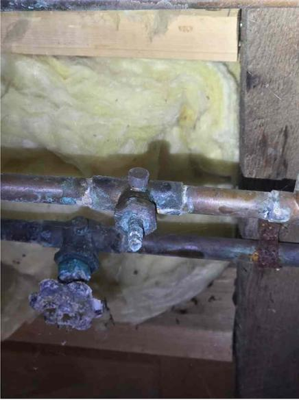
MON Noted areas of excessive corrosion on pipes or fittings. Recommend monitoring these pipes for leaks.
