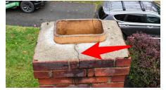
FIX Noted spalling on the chimney. Spalling is a result of water entering brick, concrete or natural stone and forcing the surface to peel, pop out or flake off.
