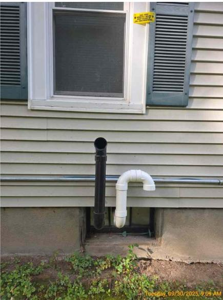
**MIN** Exterior wall penetration is missing a screen. This could allow for pest infiltration.
