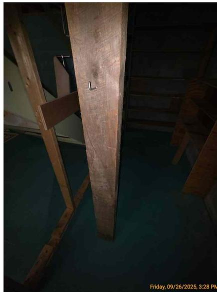
**MIN** Supports are not properly attached to the beam. This could compromise the structural integrity of the supports.
