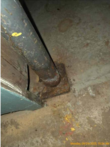
**FIX** Noted non-standard supports. This could compromise the structural integrity of the support and the floor structure above.
