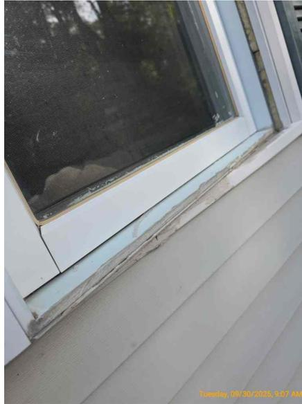
**FIX** Noted broken window. This can allow for moisture and pest infiltration.
