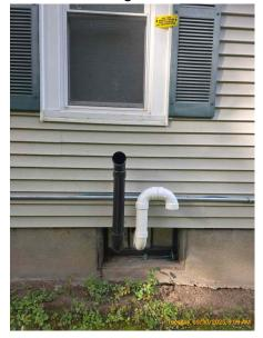
Exterior wall penetration is missing a screen. This could allow for pest infiltration.
