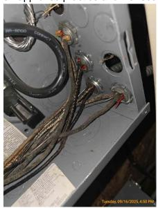
The circuitry is not completely labeled. We recommend that each circuit be identified, allowing individuals unfamiliar with the equipment to properly operate it when and if necessary.
