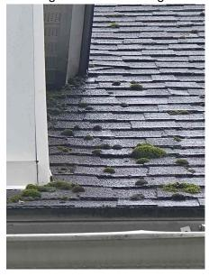
Trees are overhanging and within 10 ft of the roof surface. This could allow for moss and debris build up on the roof, or damage from abrasion.
