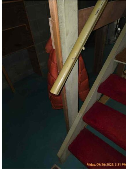
**SFTY** Noted missing guardrail on basement steps. This is a safety hazard.
