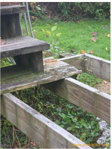
FIX Noted non-standard deck framing. This could compromise the structural integrity of the framing.
