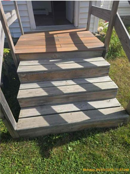
**FIX** Noted areas of rot at the time of inspection. If left as is further deterioration could occur.
