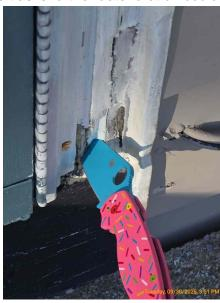
Noted high efficiency piping discharged under a window. This can allow for exhaust fumes to reenter the house through the window.
