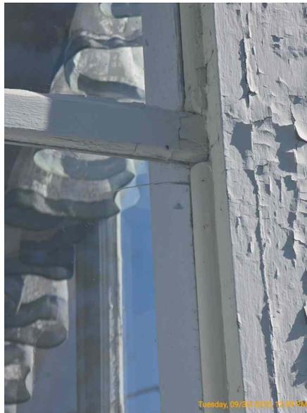
**FIX** Noted areas of rotted wood. If left as is further deterioration could occur.
