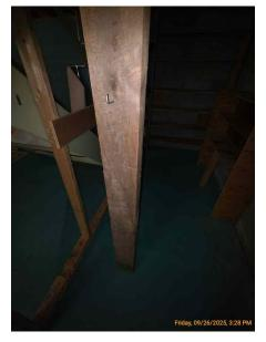
Supports are not properly attached to the beam. This could compromise the structural integrity of the supports.
