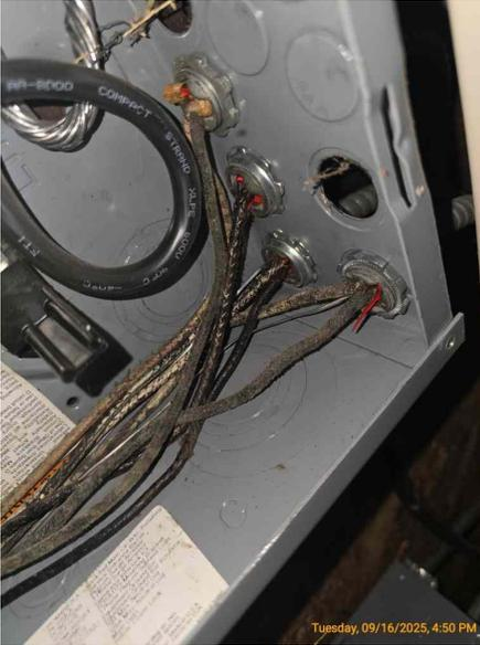
**UPGR** The circuitry is not completely labeled. We recommend that each circuit be identified, allowing individuals unfamiliar with the equipment to properly operate it when and if necessary.
