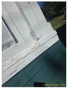
Noted deteriorated or missing window caulk at the time of inspection. This can allow for moisture infiltration.
