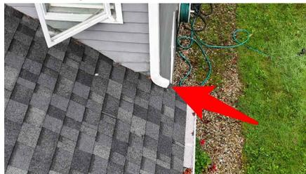
**MIN** Noted damaged gutter. This could compromise the function of the gutters.
