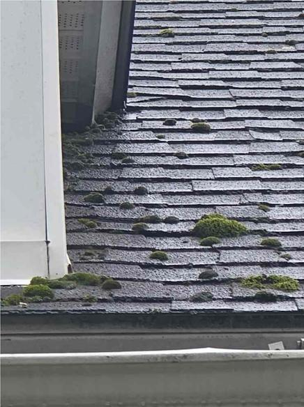
**MIN** Trees are overhanging and within 10 ft of the roof surface. This could allow for moss and debris build up on the roof, or damage from abrasion.
