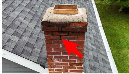
**FIX** Noted chimney crown did not extend 2 inches past the masonry. All masonry chimneys should be equipped with a crown that extends at least two inches past the masonry.
