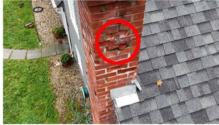
**FIX** Noted the flue is damaged. This could compromise the function of the chimney
