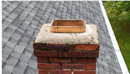
**FIX** Noted the chimney flashing was loose, deteriorated, or non-standard. This can allow for moisture infiltration.
