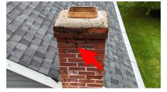
FIX Noted chimney crown did not extend 2 inches past the masonry. All masonry chimneys should be equipped with a crown that extends at least two inches past the masonry.
