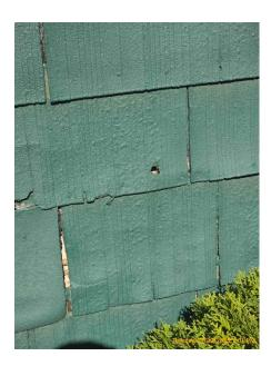
Noted areas of exposed wood in need of paint at the time of inspection. Exposed wood is more prone to deterioration.
