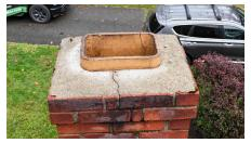
FIX Noted chimney was missing mortar in places. This may lead to moisture penetration of the chimney and eventually the roof.
