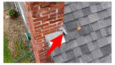
FIX Noted the chimney crown was cracked. This can allow for moisture infiltration and deterioration of the flue.
