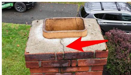
**FIX** Noted spalling on the chimney. Spalling is a result of water entering brick, concrete or natural stone and forcing the surface to peel, pop out or flake off.
